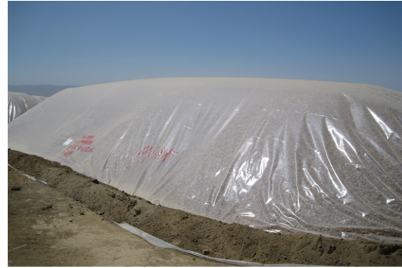
Stockpiles should be built with an even, flat top to prevent valleys where moisture can collect.
