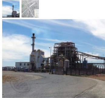
AWAITING ACTION: Greenleaf Power idled this 17-MW biomass power plant in Tracy, California, last fall when it could not compete on an unlevel playing field with solar and wind, and low natural gas prices, the basis for pricing under new PPAs. PHOTO: GREENLEAF POWER
