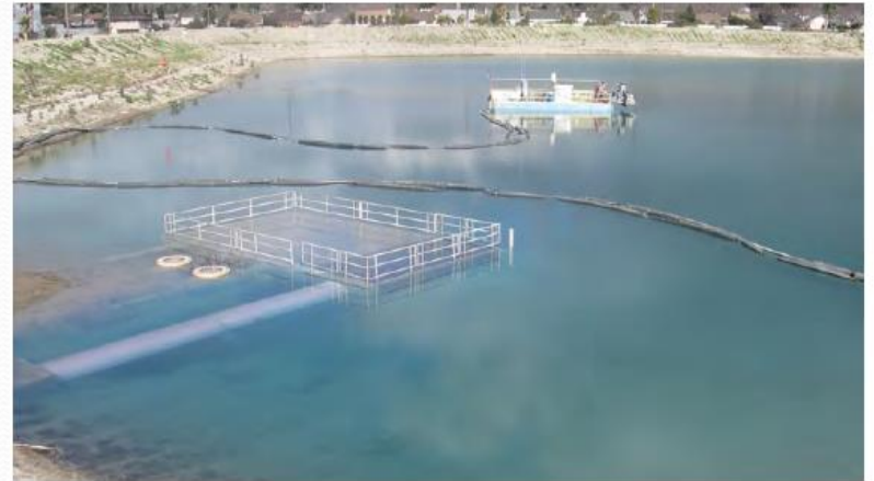
FIGURE 8: OCWD GROUNDWATER RECHARGE SITE (SOURCE: OCWD)
