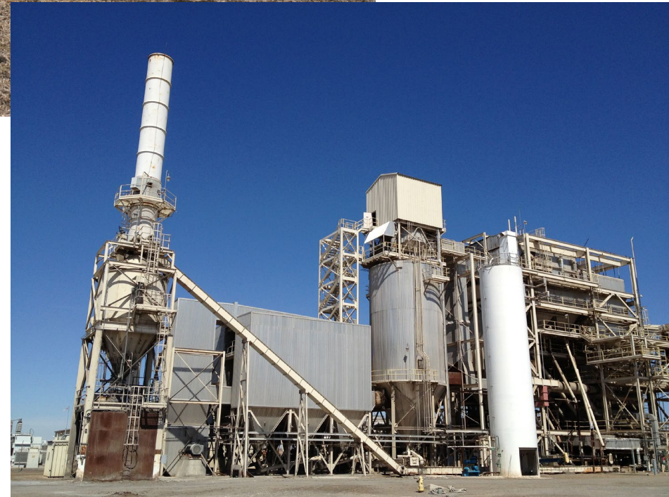
Grinding orchards for co-generation plants
